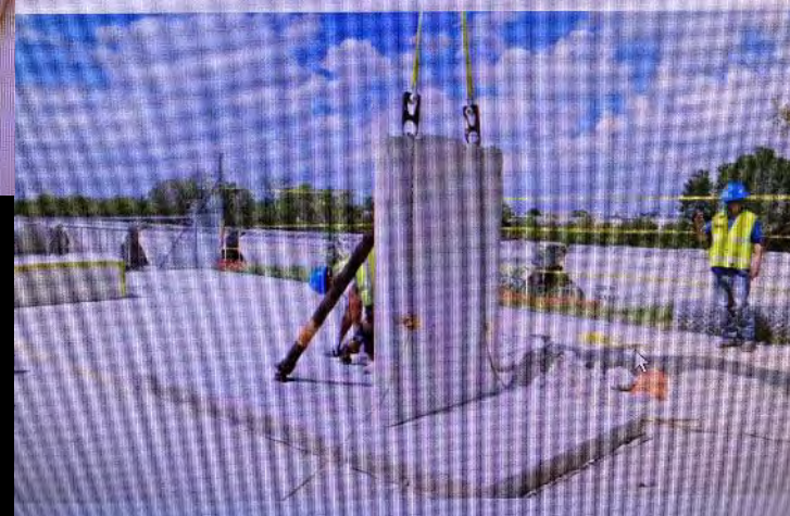
Successful Erection of 4.5 in thick panel at TCA Demo
