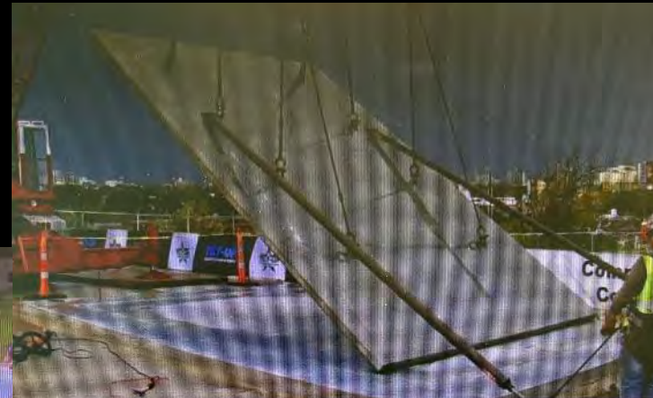
Successful Erection of 4.5 in thick panel at TCA Demo
