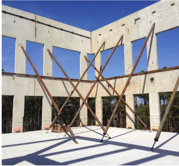
Bracing of a two-story wall panel on the Reserve at Sierra Pines Phase II building is underway.
